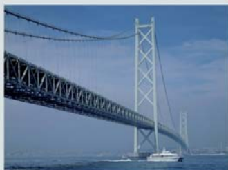
Akashi Kaikyo Bridge, Kobe, Japan
