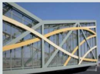
I-17 Pedestrian Bridge, Phoenix, USA
