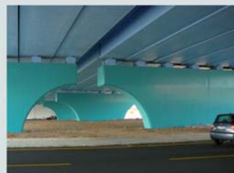
Motorway Bridge, Milano, Italy
